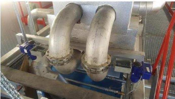
Figure 16 Bypass recuperator (still without isolation)
