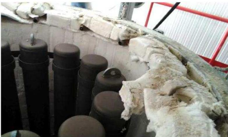
Figure 6 Insulation damage after evaporation (recording after removal of the combustion chamber lid)
